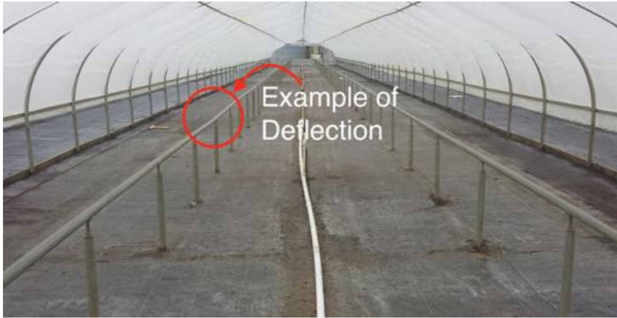
Figure 5: Rail system at Van Belle Nursery
